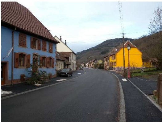
Des villages rue (ici village de Steige)
