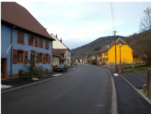
Des villages rue (ici village de Steige)
